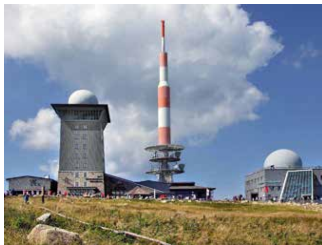
FM-radio and television broadcasting make major use of the Brocken. The old TV tower (left), the Sender Brocken, is now used as hotel and restaurant.
